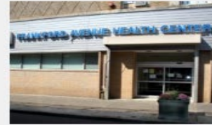
Frankford Avenue Health Center
